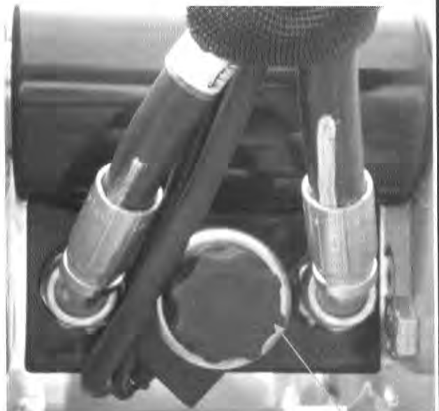
Figure 5-7. Cylinder Valve Removal
